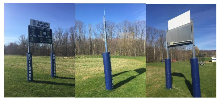
Unrepairable console and lack of replacement parts for the inner mechanics of the scoreboard were the reasons for a new scoreboard. Falling support frame of the old scoreboard is shown above.
